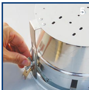
5 Adjust the clips to tightly secure the fixture and fasten with butterfly nut 将紧固件卡紧天花板后，用碟 型螺母与撑架拧紧固定
