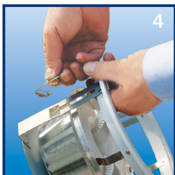
4 Install the fixture support clips 将紧固件装入外罩上撑架
