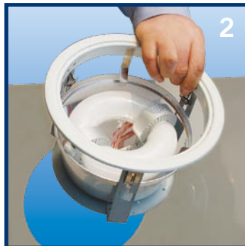
2 Insert the fixture with lamp in the ceiling panel 将装好土星灯的筒体嵌入 天花板中
