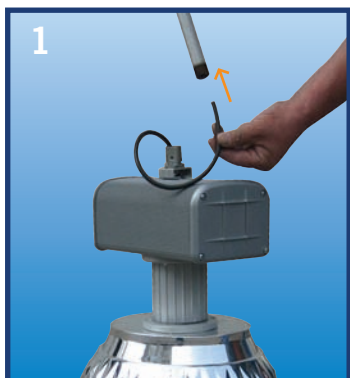
1 Thread wire through conduit 电线穿进导管
